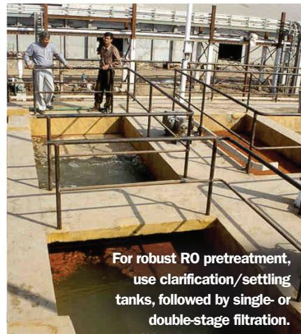
For robust RO pretreatment, use clarification/settling tanks, followed by single- or double-stage filtration.
